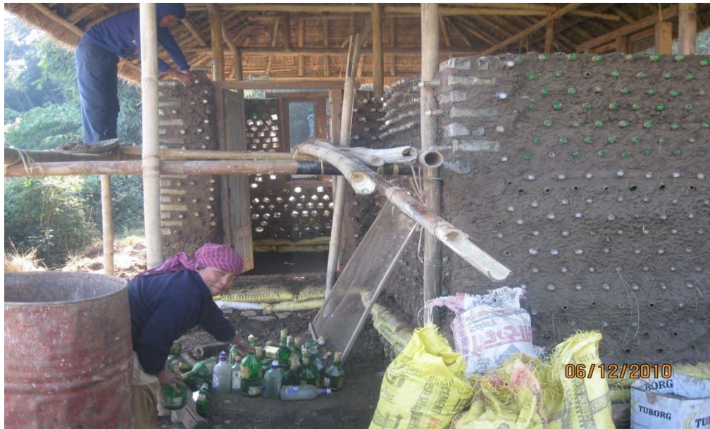
An eco house from waste liquor bottles, local clay, sand, chopped hay, local people.
